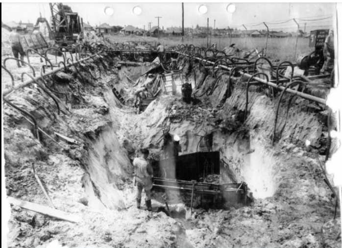
Site excavation showing flat sandy geology with de-watering in progress
